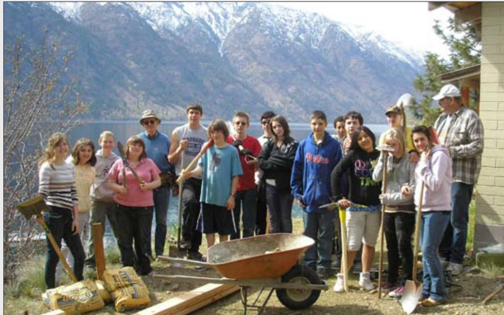
Pathfinders repair buildings, clear brush and dig holes for outhouses at Lake Chelan for the annual Teen Mission Adventure during spring break this year.
