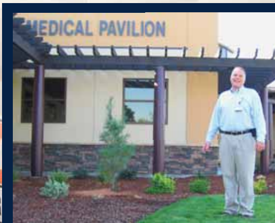
Bruce Price, Plant Services director, stands by the new Walla Walla General Hospital Medical Pavilion, which opened in the spring.
